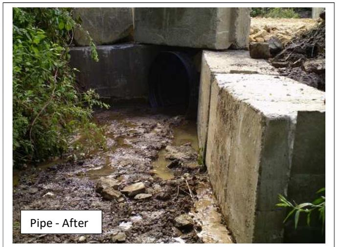
**Problem:** The existing double-pipe stream crossing was undersized and not functioning properly. Other existing crosspipes were also too small. There were wetland areas on both sides of road which caused the road base to be saturated and sink.
