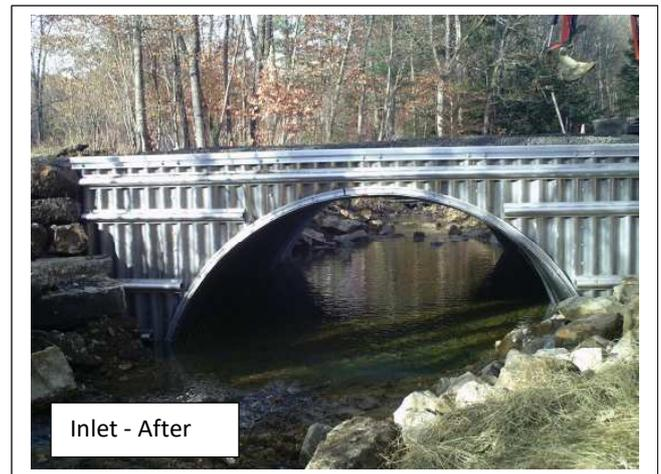
**Problem:** Existing double pipes were full of sediment, debris and were failing. Erosion was occurring around the headwall and endwall. Road ditches went directly to the stream, causing erosion.
