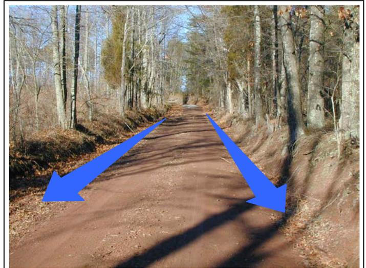
This deeply entrenched road traps drainage and is a persistent source of maintenance and erosion. Additional maintenance efforts and vehicle traffic compound the problem by lowering the road elevation further.
