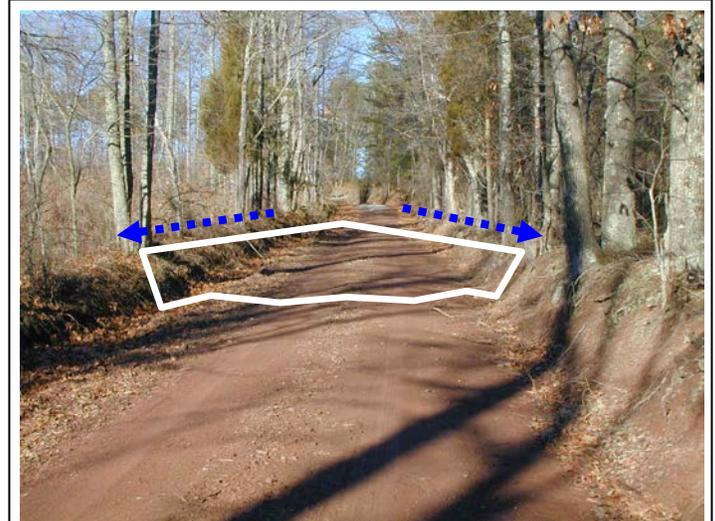
Filling the road profile here, as shown above, with appropriate center-line crown, eliminates concentrated parallel ditchflow and allows water to sheet flow off the road into surrounding terrain, reducing the erosive force of “hungry” water and saving scarce maintenance funds.
