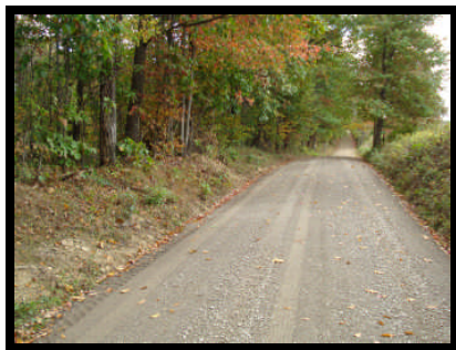
“Dirt & Gravel Road Project”
