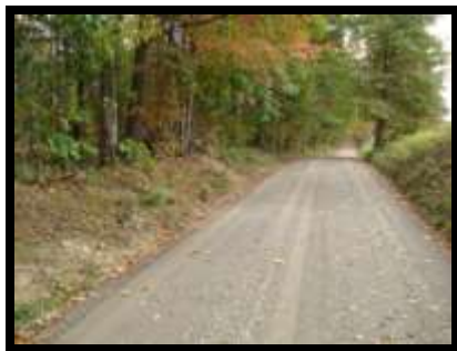
“Dirt & Gravel Road Project”
