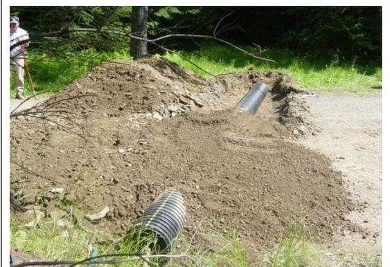
This shallow pipe is being covered with fill. The fill will be ~18 inches above the existing road over the pipe, and taper out for 50+ feet in both directions
