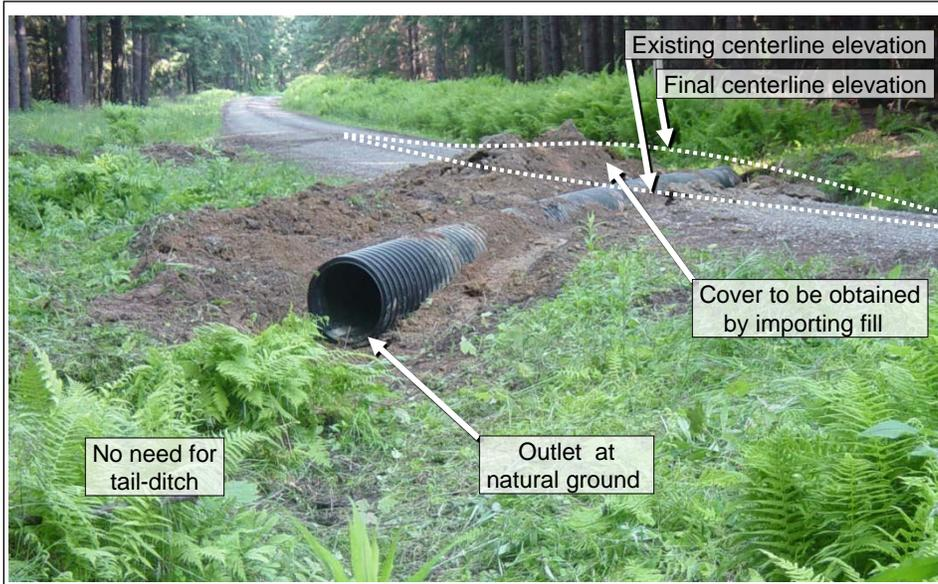
The crosspipe shown here is partially installed. Notice that the outlet of the pipe is at the elevation of the existing ground, no outlet trench or tail-ditch is required. Also notice that the top of the pipe is actually ABOVE the existing road surface. The minimum of 12 inches of pipe cover will be obtained by importing cover. When completed, the cover will create a gradebreak over the pipe.
