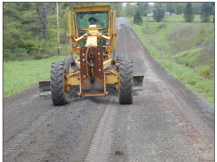
**Figure 3.** The material is knocked down (above) leaving the road with a high flat center (far left).
