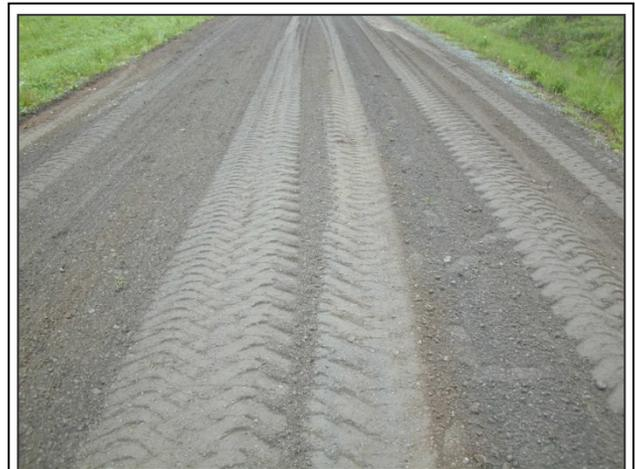
Figure 5. Here the grader was used to partially compact the groomed road. Slightly offsetting the wheels on an articulating grader allows the operator to compact twice as much area with each pass.
